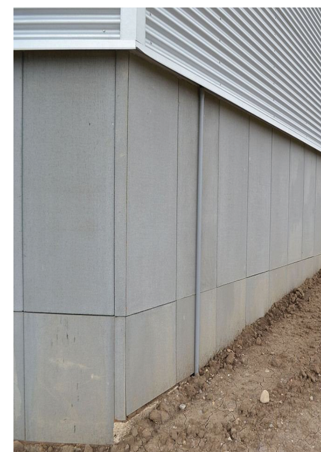
Wallguard - Concrete faced insulated perimeter wall.
